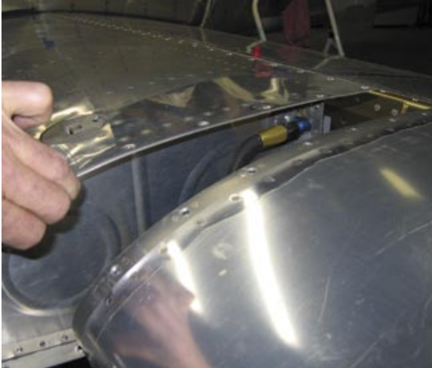
The main tank is reinstalled on the wing, with the aux tank fuel line visible on the right.
